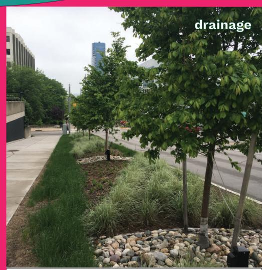
A bioswale is a long, channeled depression or trench that receives rainwater runoff and has vegetation and organic matter to slow water infiltration and filter out pollutants.
