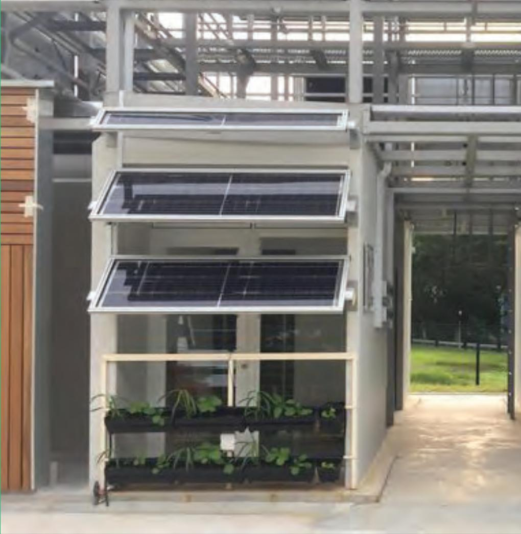
Productive facade systems are used for energy and food harvesting. Facade elements that enhance indoor daylight conditions, shading, and thermal performance, and wind permeability and productivity benefits (food, alternate energy source or air-conditioning).
