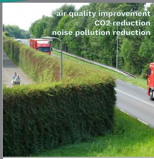
Greennoise barriers include all noise abatement/mitigation structures that form a part of a road system, including vertical, cantilevered/curved barriers and noise enclosure including in the design vegetation adapting to the surrounding environment, at grade or on elevated structures.
